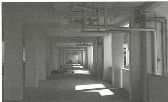
Roof podium, People's Park Centre, Singapore, 2019
