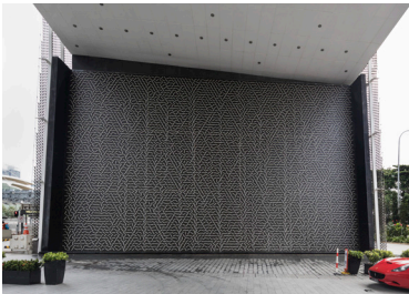
Tipping Wall Ned Kahn 2011 Marina Bay Sands Integrated Resort
