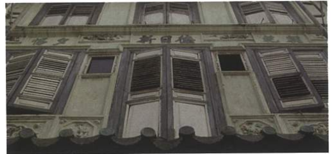
Baba House • facade before restoration
