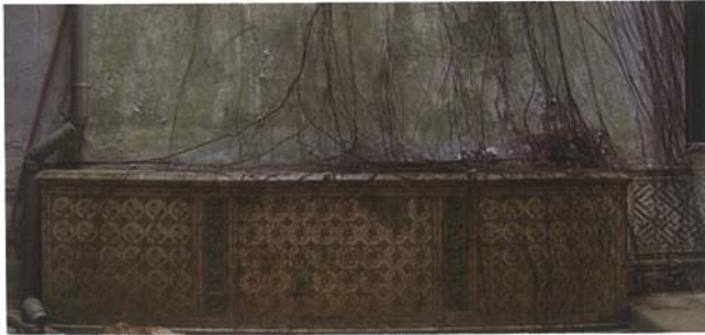
Baba House • airwell area before restoration
