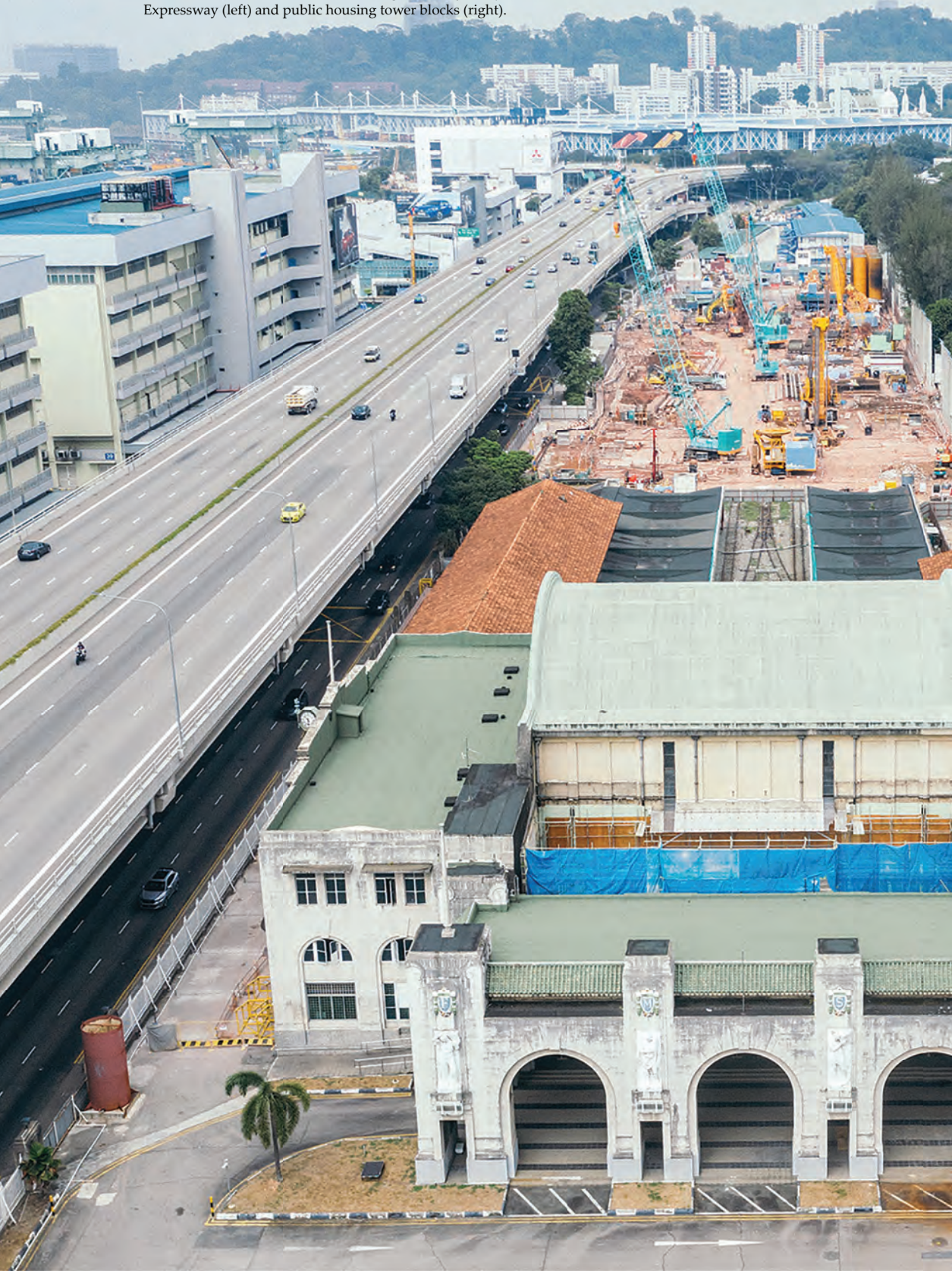
3.4 The station is located between the eight-lane Ayer Rajah Expressway (left) and public housing tower blocks (right).
