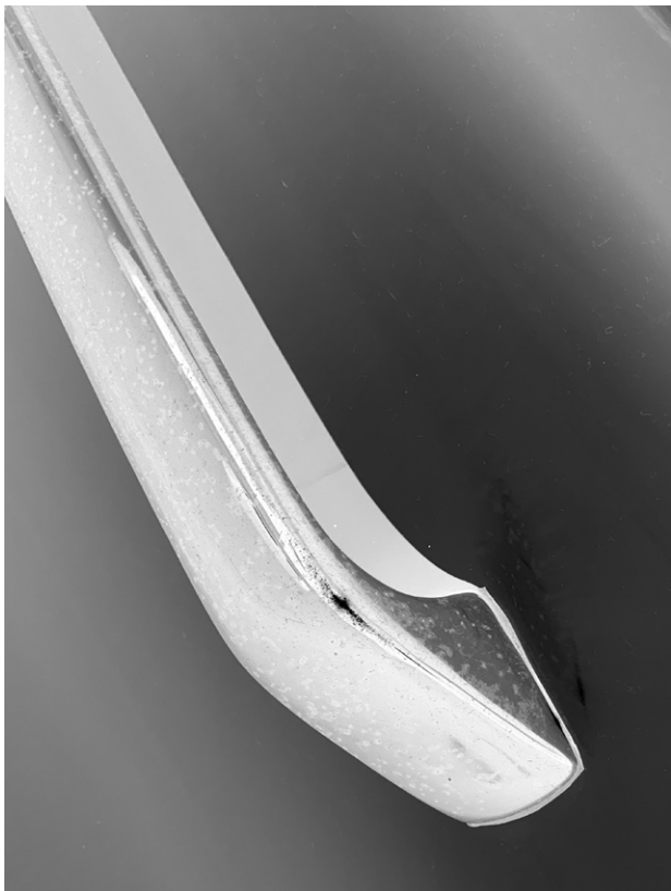
Water stains and scaling on grab bar
