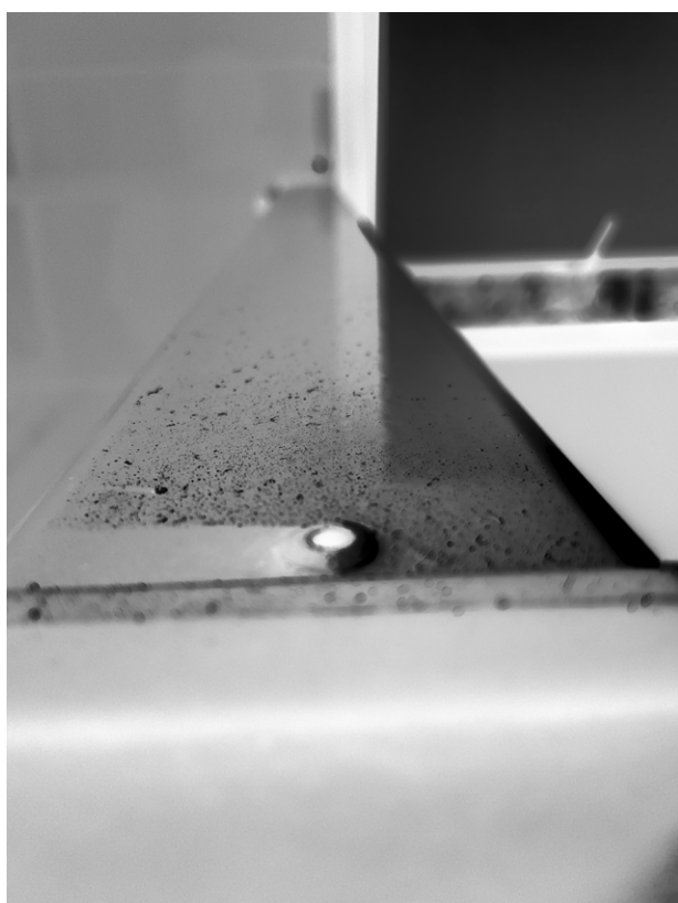
Dust particles atop sliding screen channel
