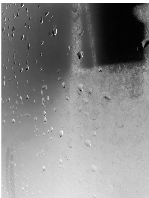
Water stains and droplets on acrylic screen
