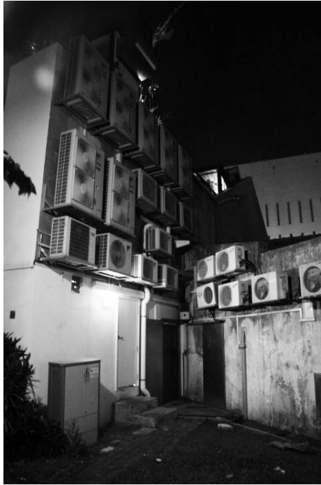
11: Backdoors leading to hidden corners.
