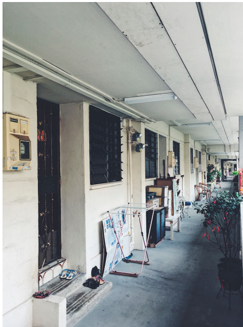
Figure 5. The 'access balcony' or common corridor, 2017 (photograph by Lin Derong).
