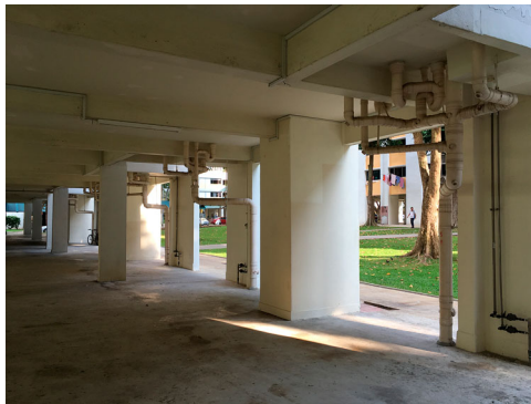
Figure 8. The spatially porous void deck, 2017 (photograph by Lin Derong).
