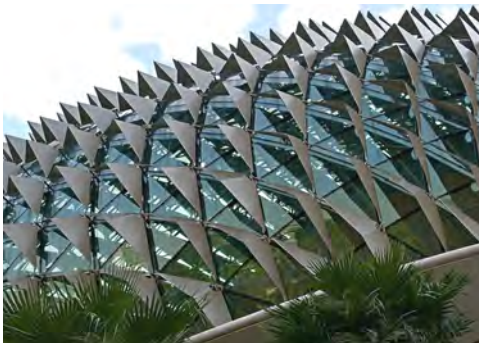
August 2008. fig. 4.1: Sun shading device of the Esplanade. http://www.architecture.about.com/cs/greatbuildings/a/esplanade.htm (accessed 5th August 2008)
