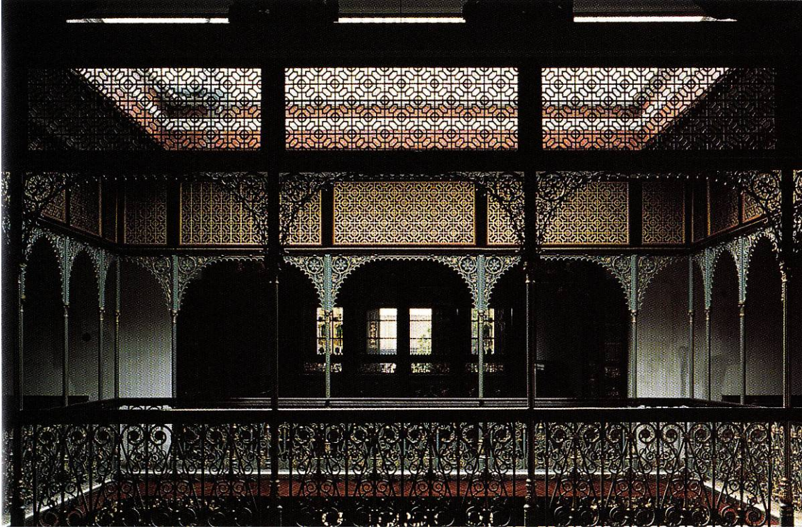
15 Delicate cast-iron woven onto columns and balusters.
