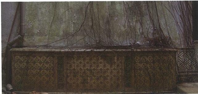
Baba House • airwell area before restoration
