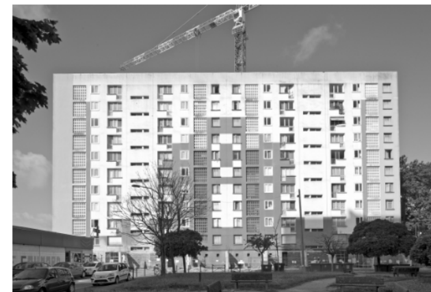
Old Facade of Transformation of 530 Dwellings
