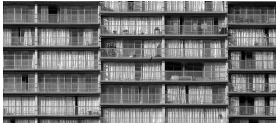
Facade of Transformation of 530 Dwellings
