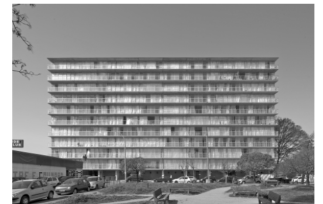
Renovated Facade of Transformation of 530 Dwellings
