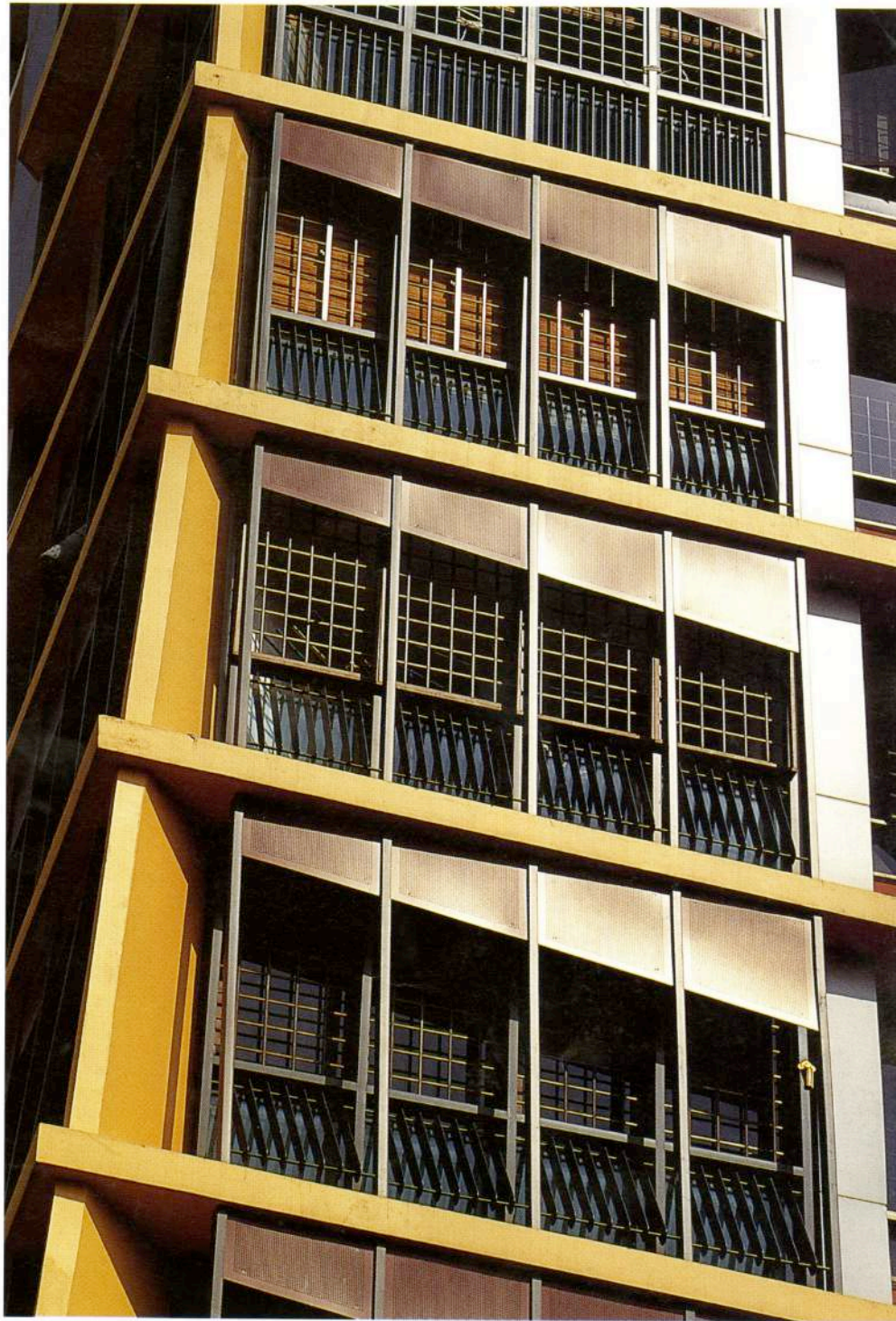
Above A frontal layer of lattice-like balconies are vertically mediated by a defiant dividing wall and sliced horizontally by rhythmically placed fins both painted yellow
