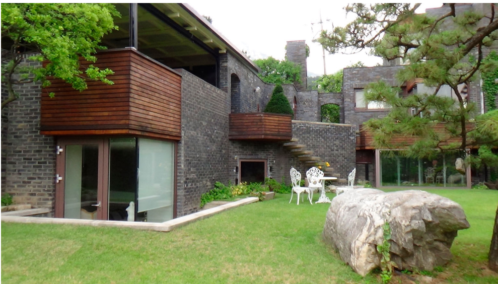
Figure 10. Cedar timber framework on the exterior of Ch'angamjang (source: the Author).
