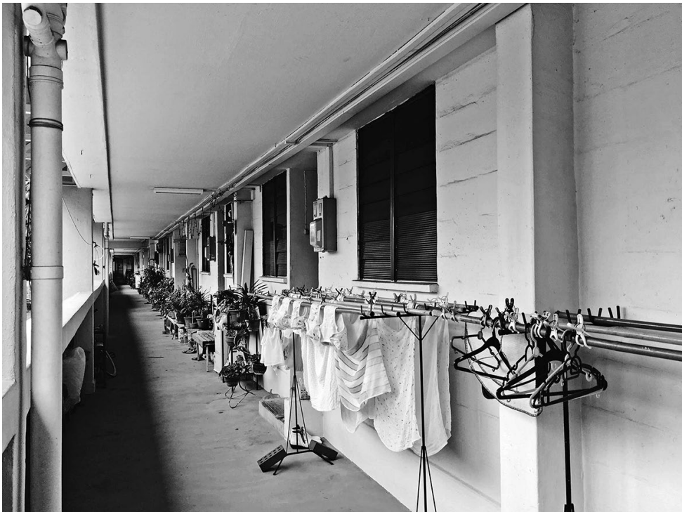
Figure 3.2 The common access balcony or corridor of a HDB flat. Photo: Lin Derong, 2017.
